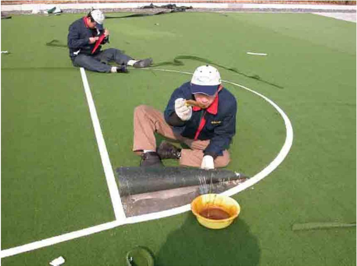
**17<sup>th</sup> step: glue on the foundation on the edge of penalty area and the lawns, clapped them together after air-dry.**
