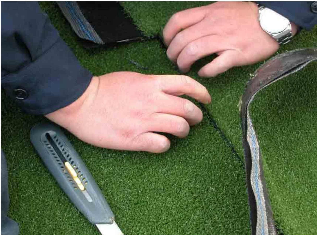
**Tenth step: joint and cut the redundant lawns between rolls.**
