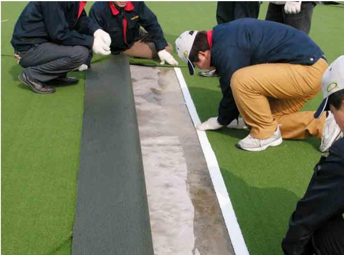
**16<sup>th</sup> step: glue the joint between the white and green lawns (width is 15cm-20cm), clapped them together after air-dry.**
