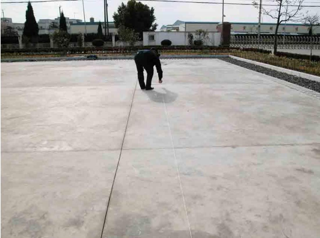
**First step: Based on the basketball court to identify the location of all the white line and later snap the ink and carpenter's sink marker.**
